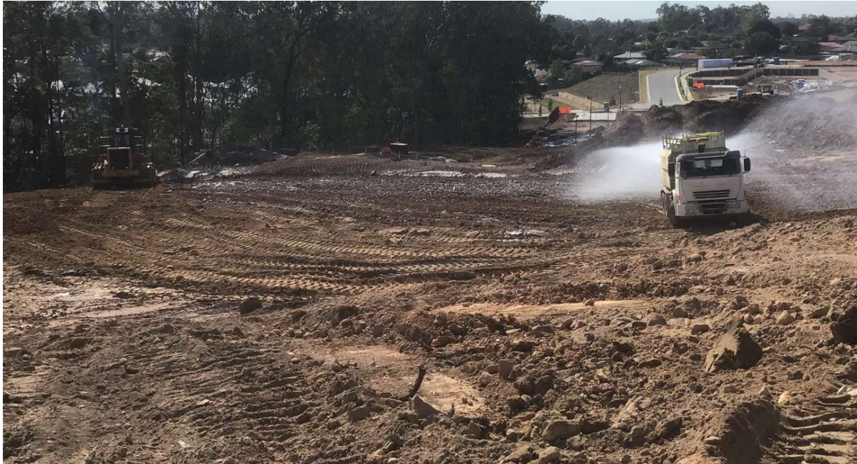
Site Image 1 – Filling Operations in Progress
