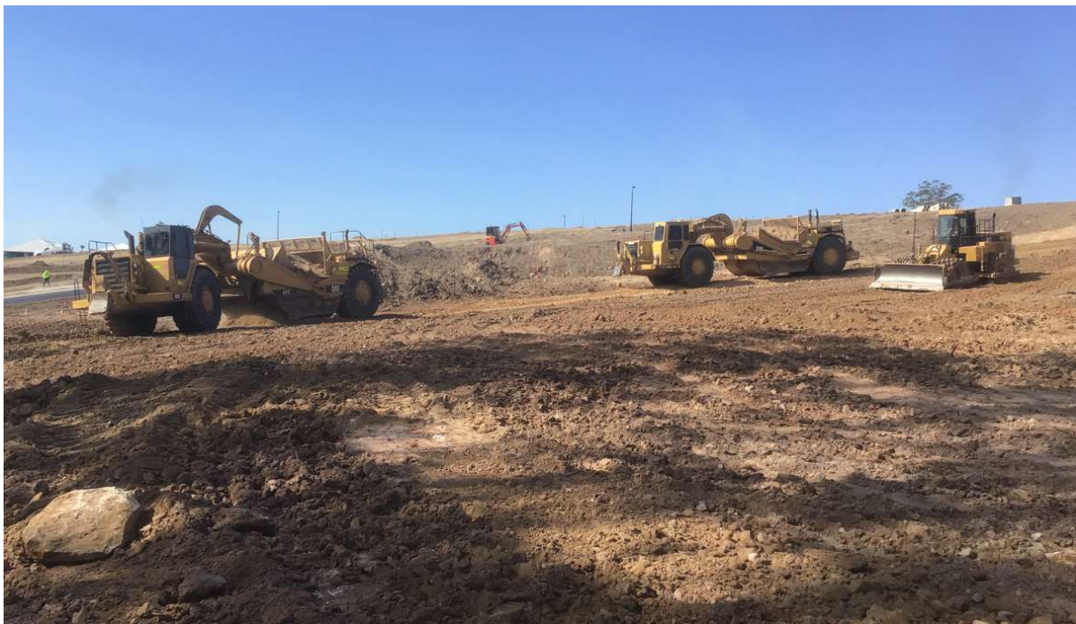
Site Image 2 – Filling Operations in Progress
