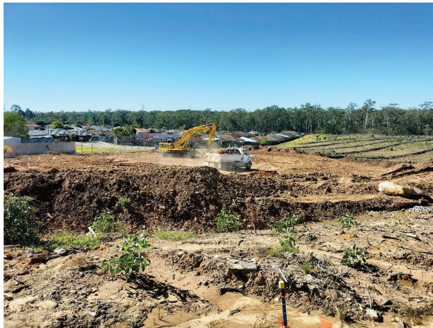
Site Image 2 – Filling Operations in Progress (19/07/2023)
