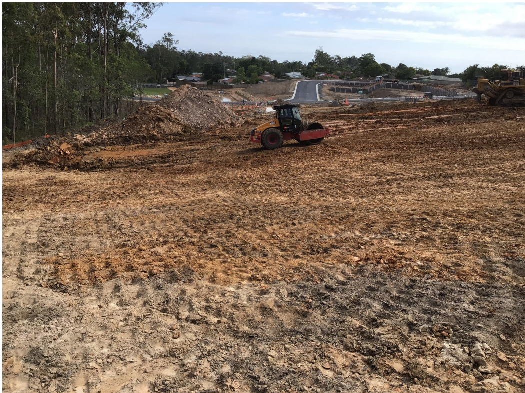
Site Image 2 – Construction in Progress (14/12/2022)
