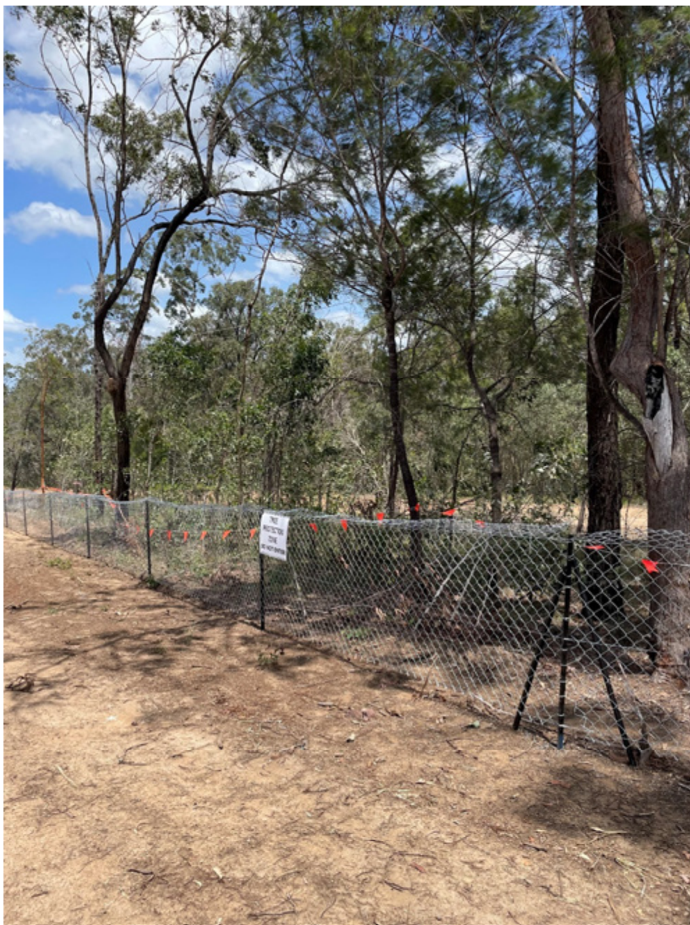
Photo 1: Evidence of temporary koala exclusion fencing erected at the impact site.
