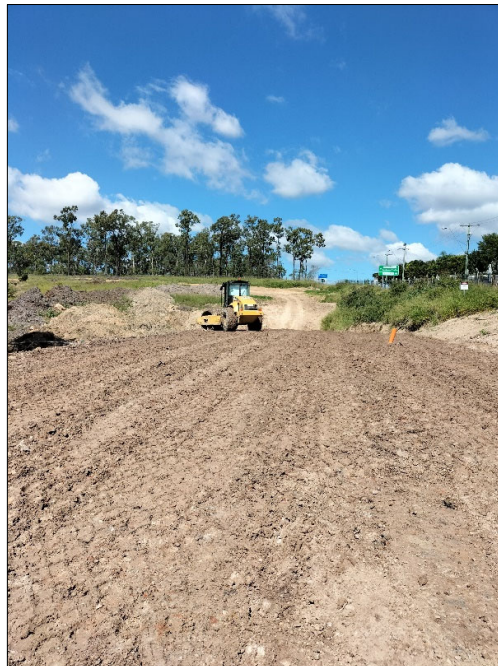
Figure 2 – Pad Foot Roller working material along Road 02.
