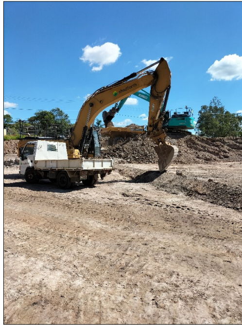
Figure 3 – Excavators loading material to be removed from site.
