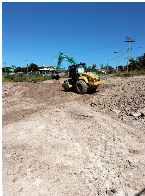
Figure 4 – Excavator placing fill with a Pad Foot Roller working the strip.
