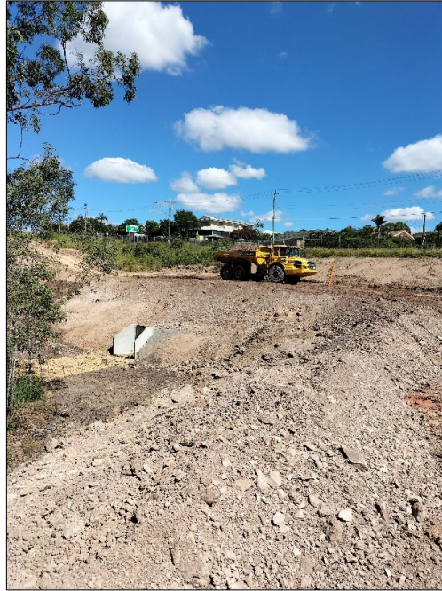
Figure 1 – Moxi trucks removing excess material offsite.
