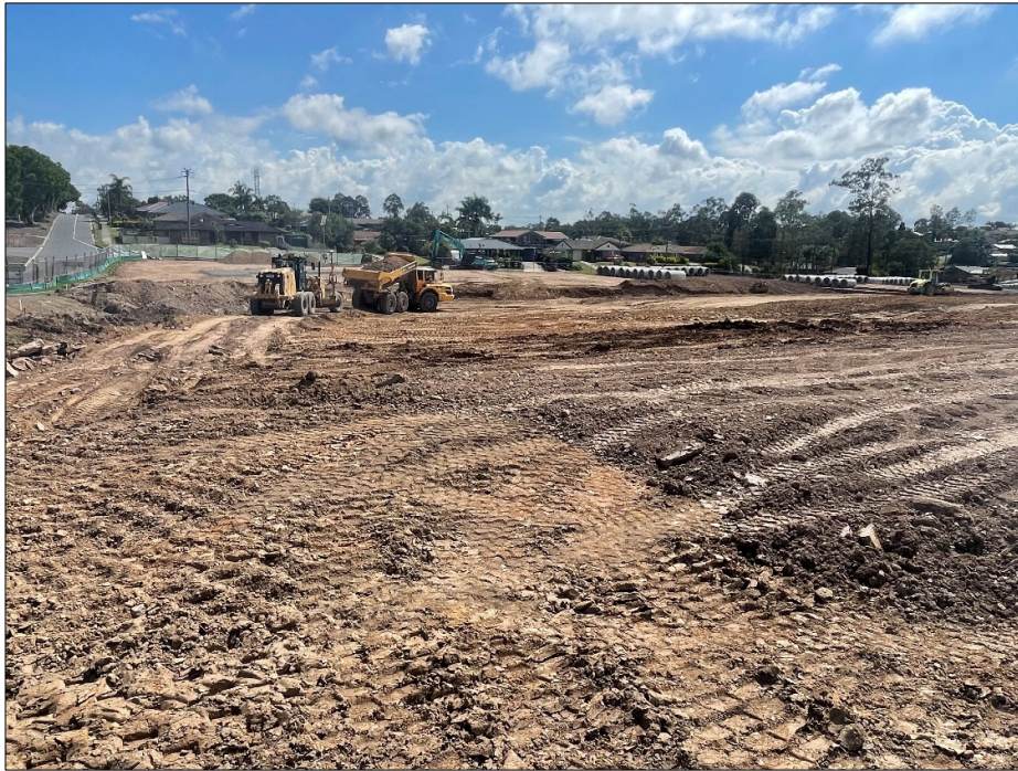
Figure 5 – Fill being placed, grader trailing behind and spreading fill out. (Taken: 21.10.2021)
