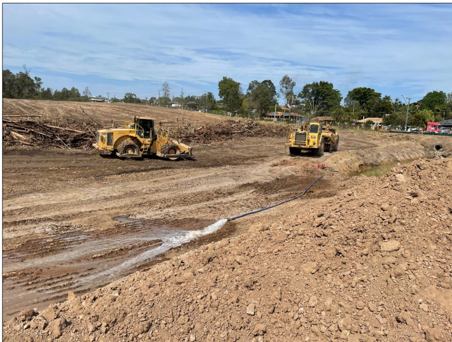
Figure 5 – Layer being cut back of excess material with a belly scraper, water being drained from nearby (Taken: 21.10.2021)
