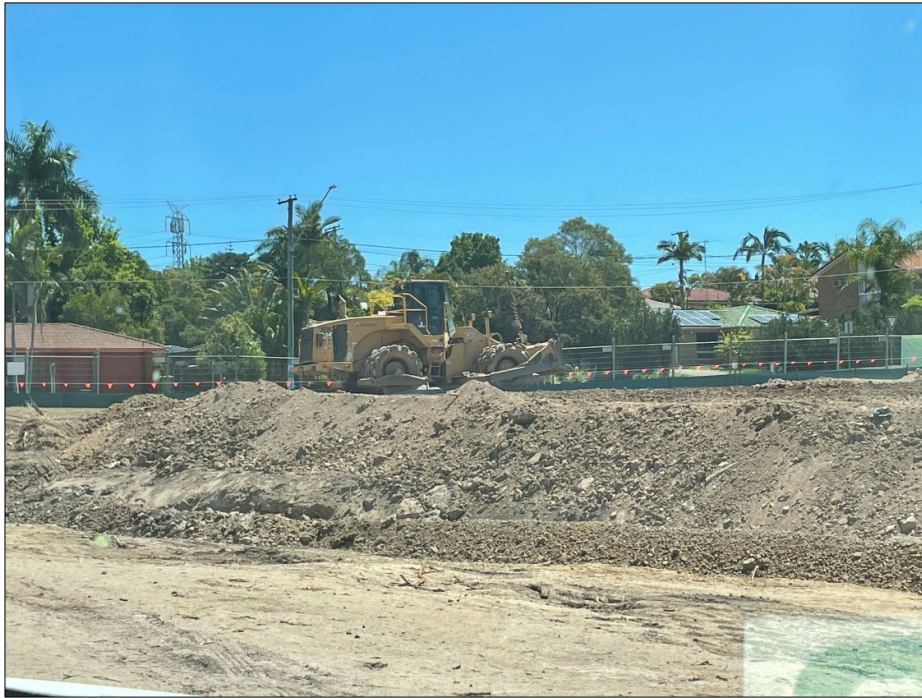
Figure 5 – Test rolling being completed. (Taken: 21.10.2021)
