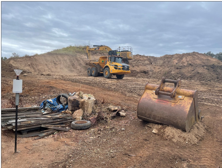
Figure 4 – Excavator loading moxy with cut material. (Taken: 30.09.2021)
