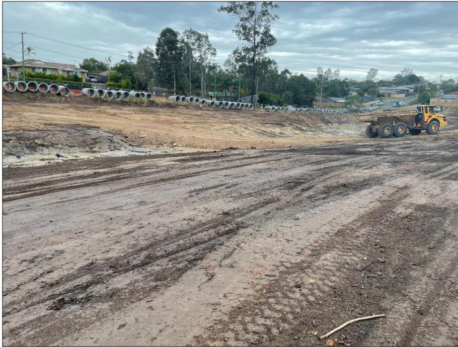
Figure 1 – Moxy removing cut material and stockpiling elsewhere. (Taken: 30.09.2021)
